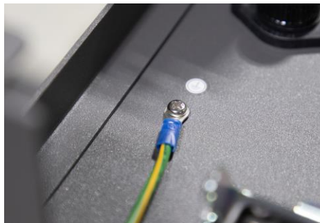
Figure 22: Securing the ground wire with control box
